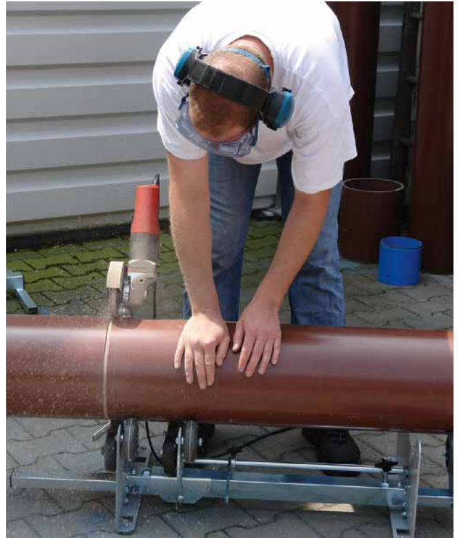
Cutting to length and simultaneous chamfering of the pipe
